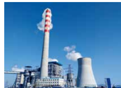
山东枣庄 350 MW 超临界多边形炉膛循环流化床锅炉 350 MW Super-Critical CFB Boiler with Polygonal Furnace in Shandong Province
