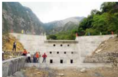
泥石流防治工程 Engineering mitigation for debris flow hazard (check dam)
